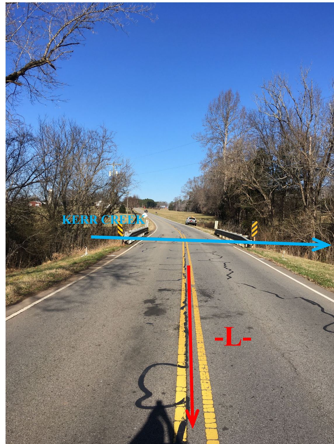
Looking North towards End Bent 2
