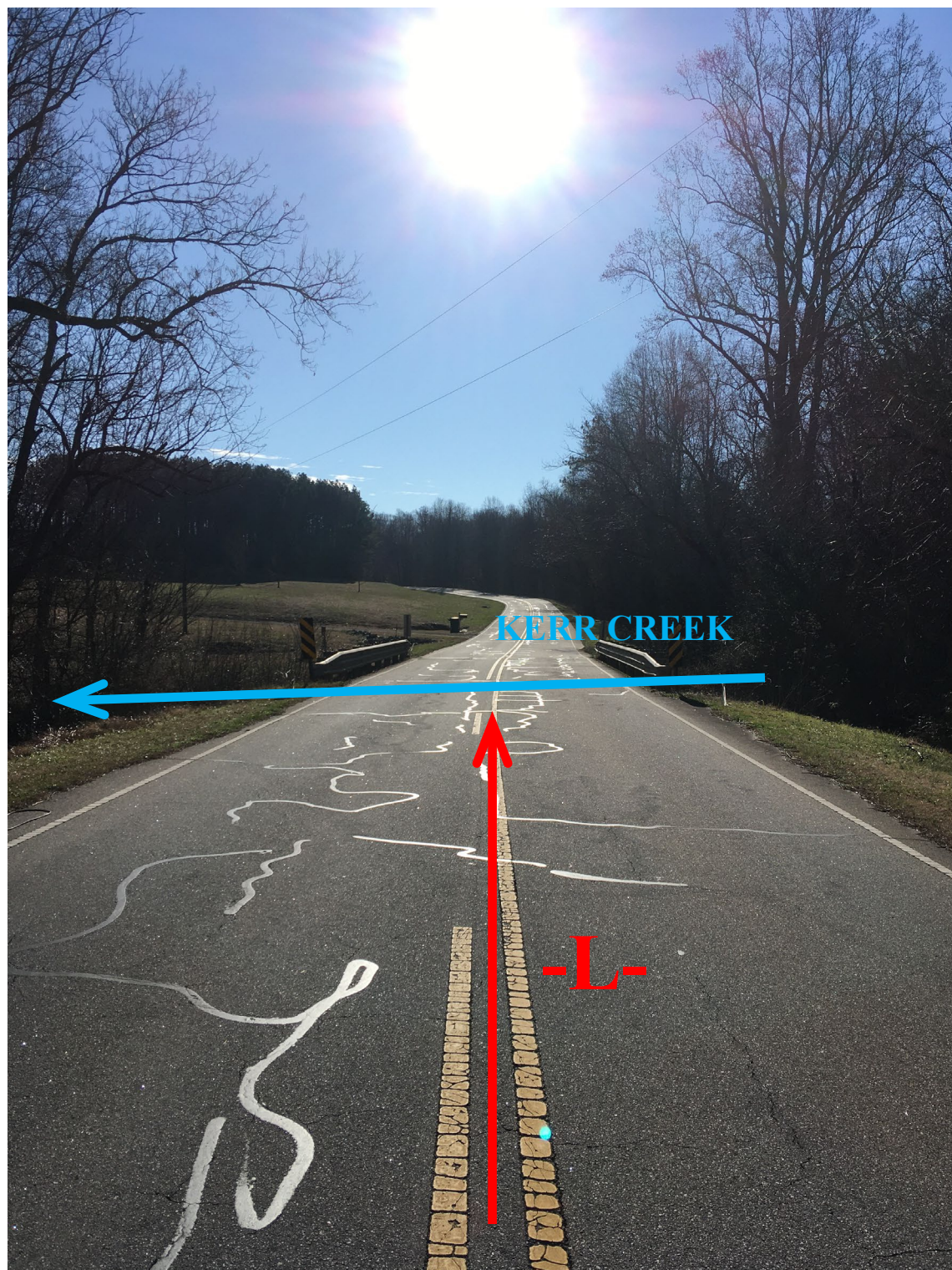
Looking South towards End Bent 1
